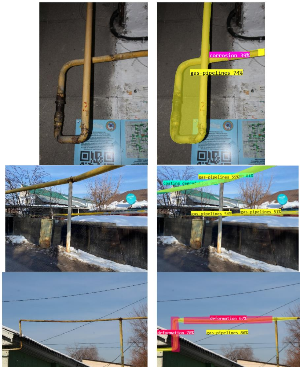
Fig. 3. Example Defect Detection Results (YOLOv11-M)
