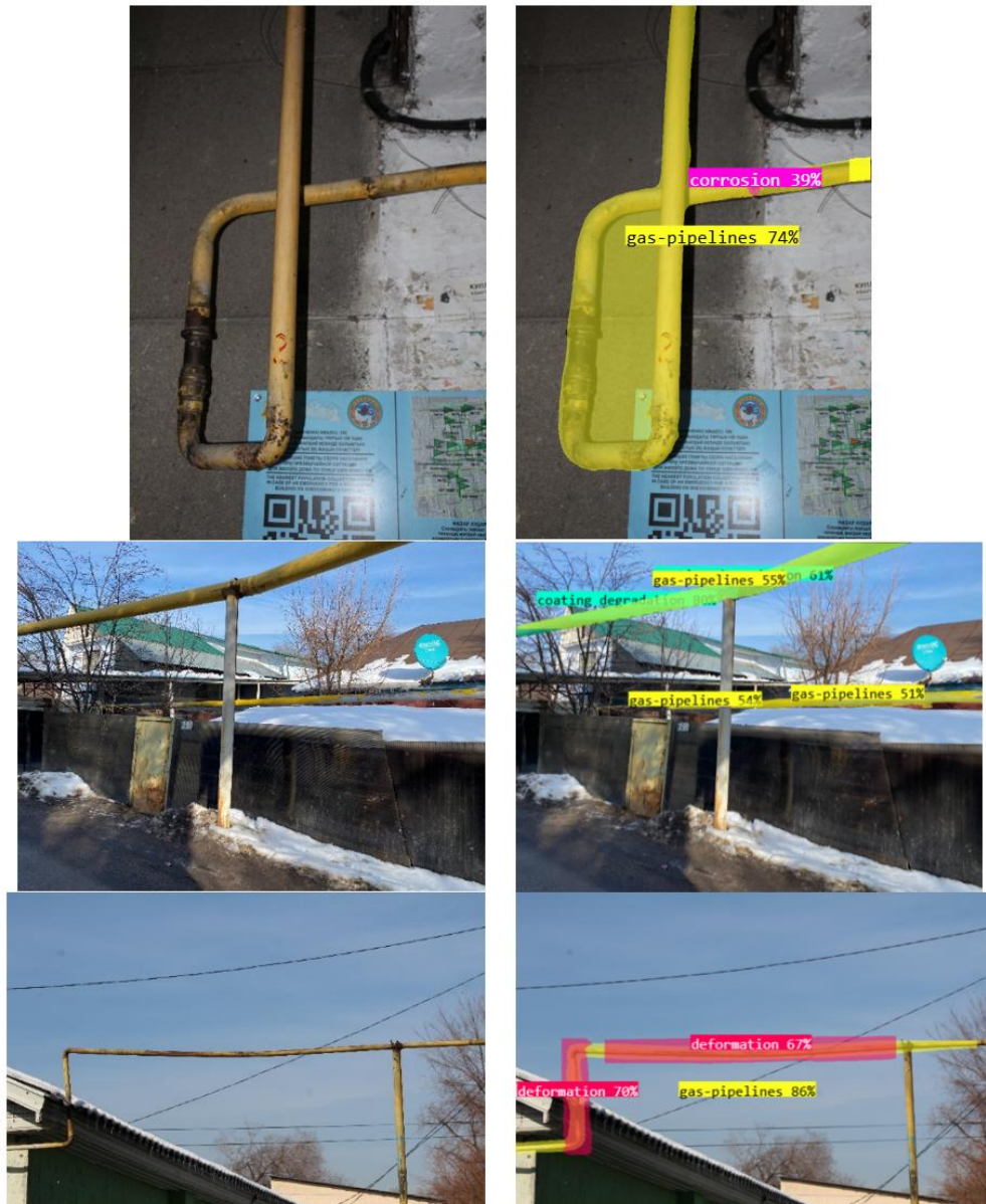
Fig. 3. Example Defect Detection Results (YOLOv11-M)
